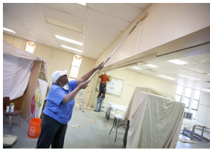
Deb Harris pitching in to help with community center improvements.
